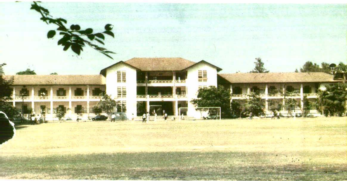
The oldest existing building of Sakon Nakhonrajavidyalaya University at Prasannit campus
